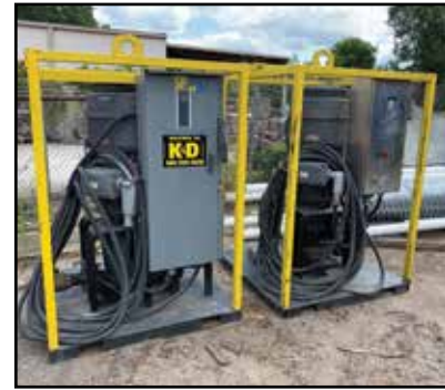
(2) INGERSOLL-RAND 60-HP Skid-Mounted Pumps
